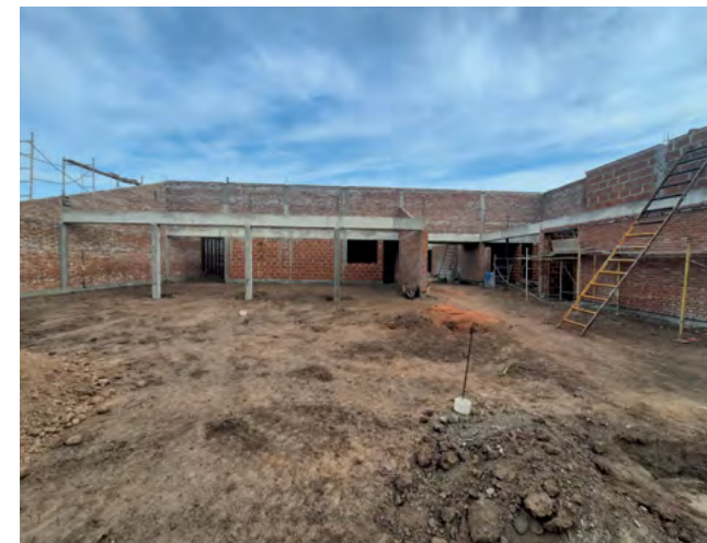
Construction work on the Casita del Niño Rincón del Sol headquarters.
